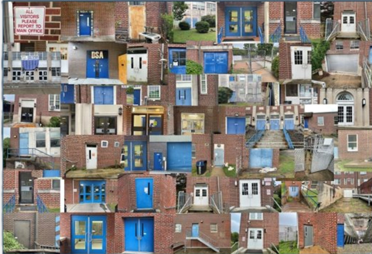
68 Exterior Doors to Secure
