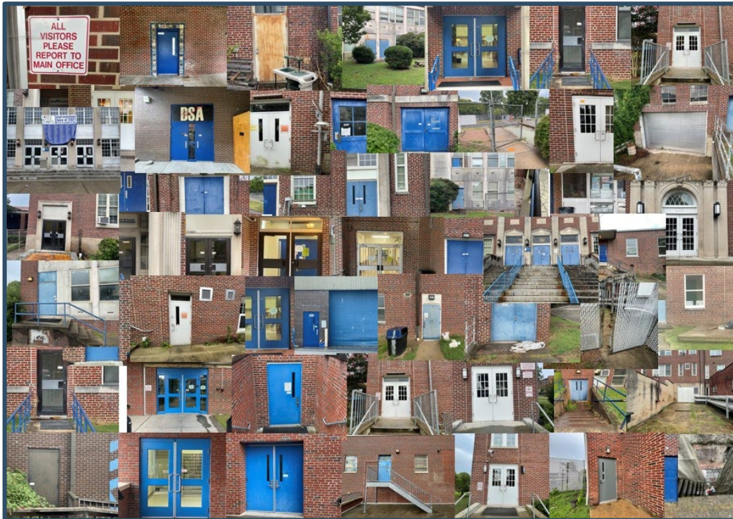
68 Exterior Doors to Secure
